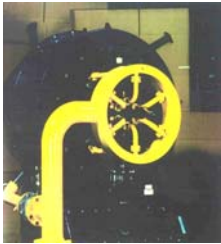
Gas piping system with gas distribution ring
